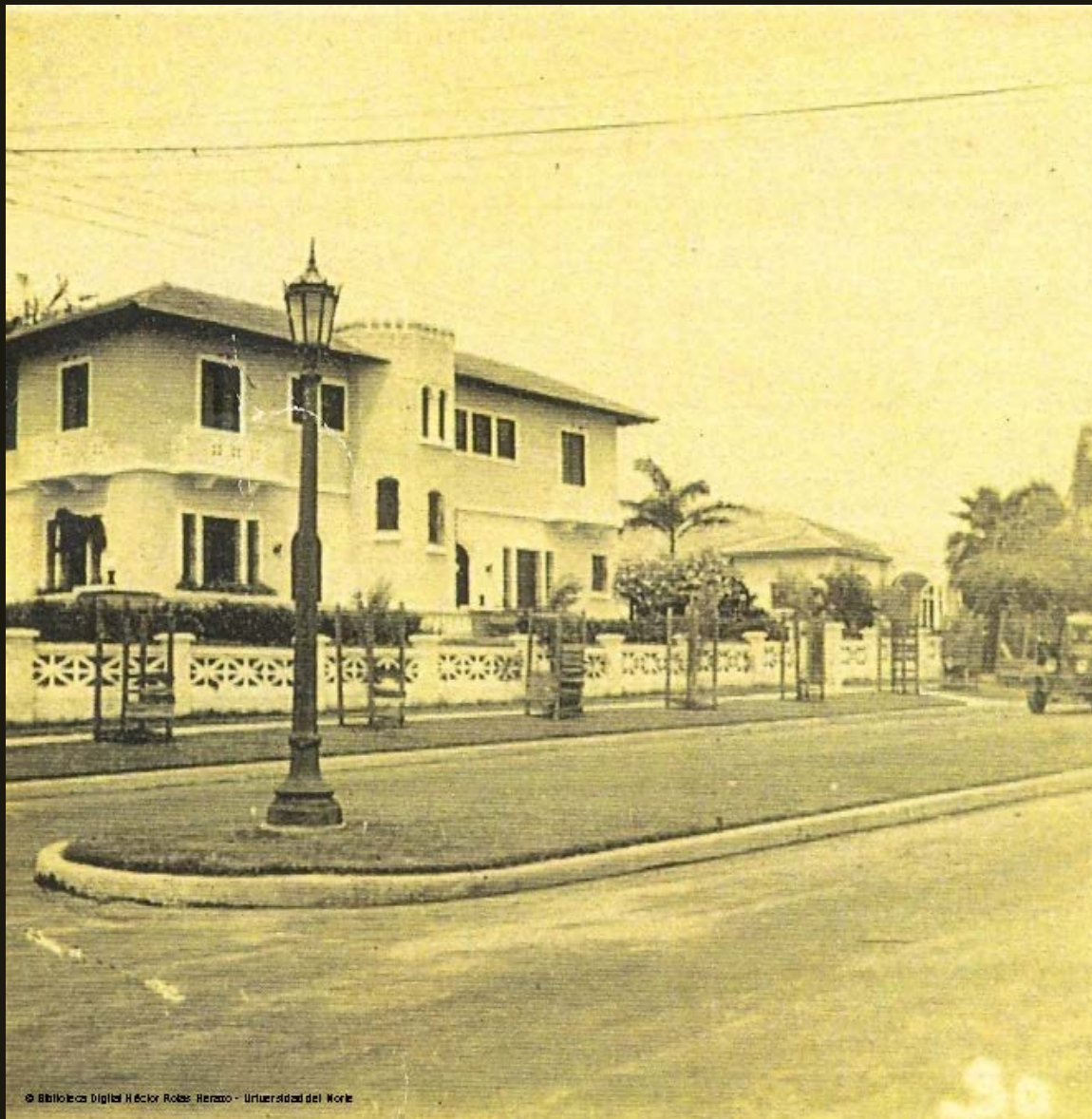
Picture N° 28. Houses at "El Prado" neighborhood.
