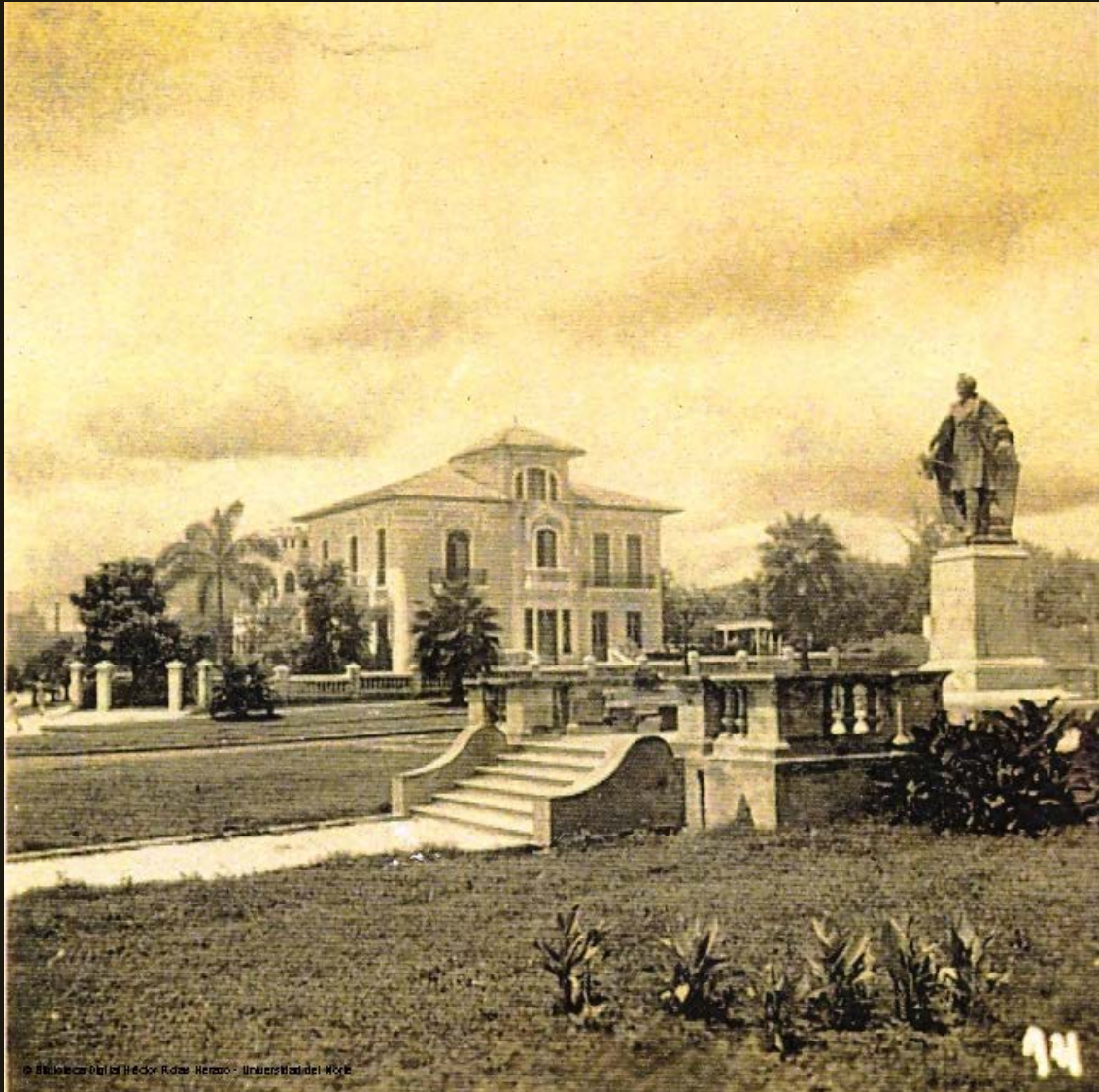
Picture N° 39. Houses at “El Prado” neighborhood.
